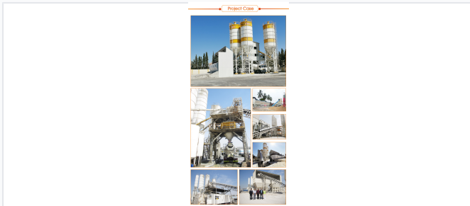
The batching plant in operation at a large-scale infrastructure construction site.
