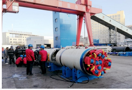
A heavy-duty machine prepared for trenchless underground construction.
