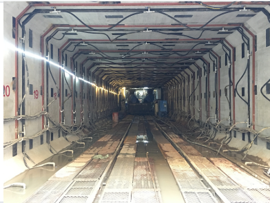
The machine performing precise excavation within a finished tunnel segment.
