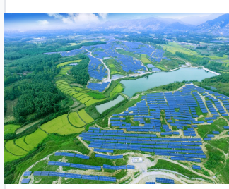
Photovoltaic modules arranged in rows across a terraced landscape.
