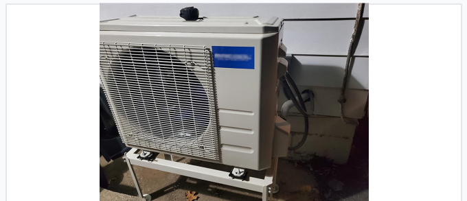
Elevated design protects the condenser unit from ground debris, moisture, and snow.
