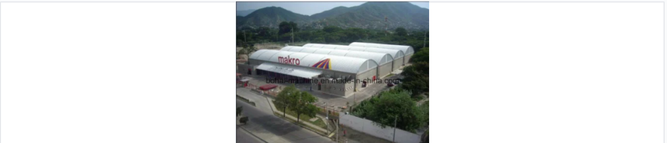
Example of a completed large-span structure produced using this roll forming technology.
