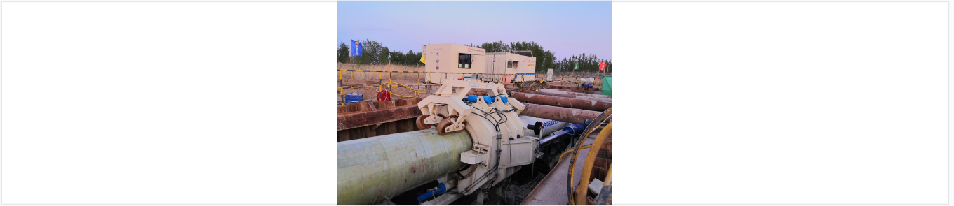
Operational setup showing the pipe handling and thrusting mechanism at a construction site.
