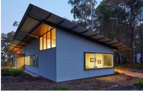
Example of finished corrugated metal sheets applied to a modern residential roof design.
