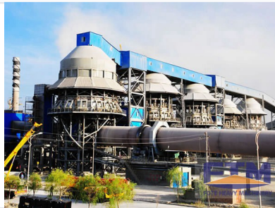
A detailed view of the cement grinding station, showcasing the rotary kiln, cyclone preheaters, and integrated support structures for clinker processing.
