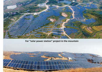
Successful solar power station projects from "QIXING"
