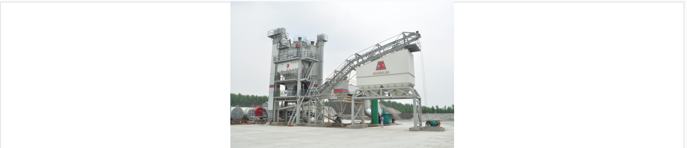
Stationary asphalt production system showing the mixing tower and aggregate supply components.
