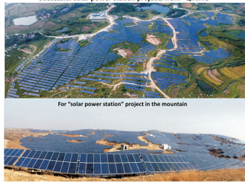
Successful solar power station projects from "QIXING"
